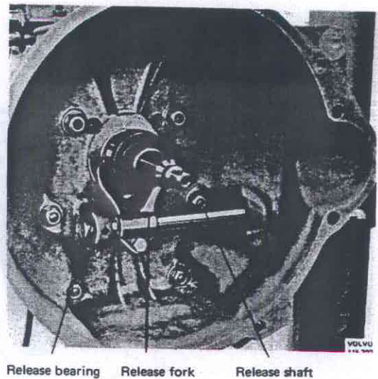
Fig. 41-5. Installing the clutch
